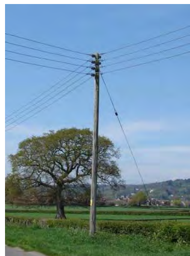
Figure 4 Typical 400 V overhead line open wire (can also be insulated and bundled)
