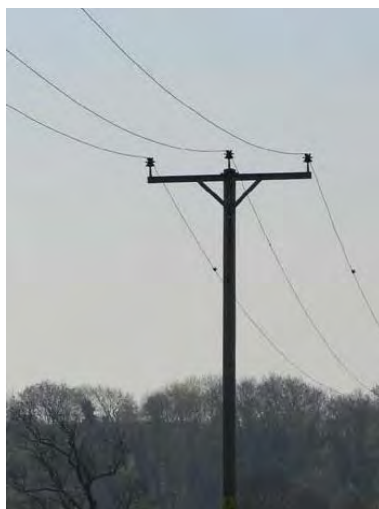
Figure 3 Typical 11 kV overhead line single-circuit line (can also be double-circuit)
